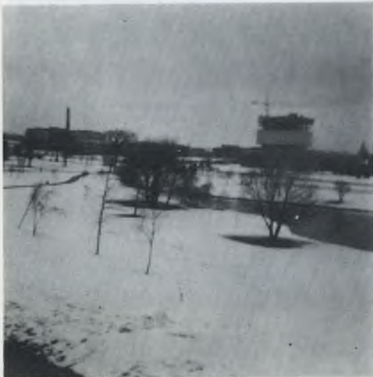
A winter view of the University of Waterloo campus.
